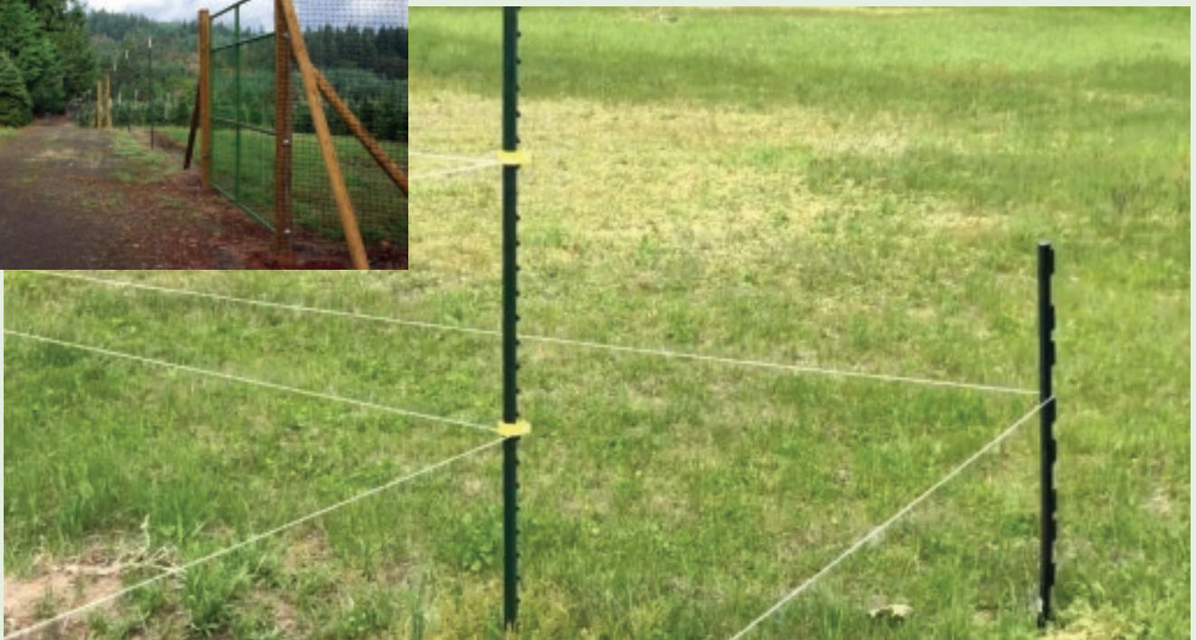
FIG 5 – Two-tiered (or 3-D) electric deer fences exploit deer’s poor depth perception to exclude deer. Photo: Brian Dooley, dooleyhomestead.com.
